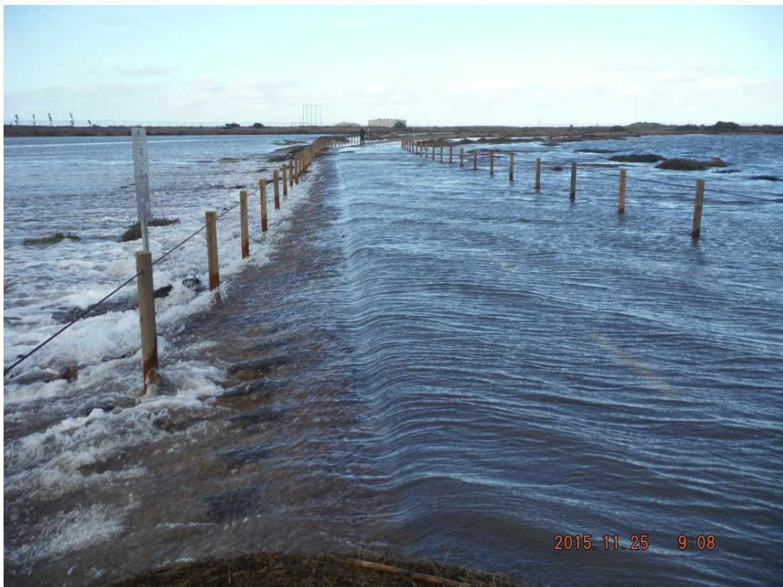
Figure 3-2. Overtopping of the Bikeway on 11/25/2015
